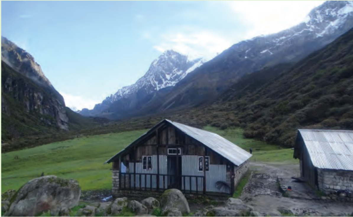
Fig: Overview of Thangsing Log house
